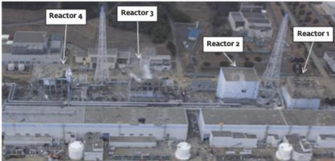
Figure 3.4.: Photograph of the four units of FDNPP I after the accident. Whereas the reactor building of Unit 3 and 4 and the upper part of Unit 1 were destroyed by hydrogen explosions, the reactor building of Unit 2 looks intact, apart from the opening of the so-called blowout-panel. [69].
