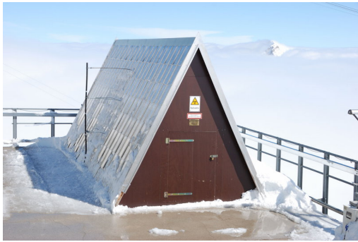
(a) Experimental shed at the UFS in an altitude of approximately 2660 m
